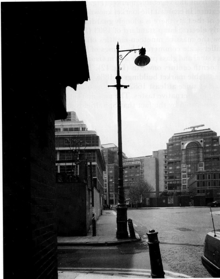
Fig. 11 Electric Lamp Standard, Brushfield Street, Spitalfields, Tower Hamlets, London. Erected in 1903 for Stepney Borough Electricity Supply RCHME Crown Copyright
